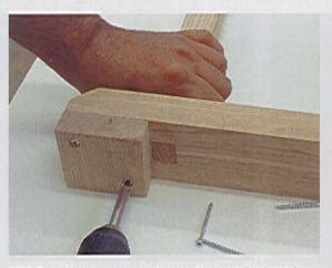
STEP 7 To save wear and tear on the lower horizontal supports, install sacrifice pads. These are 3"-square by 1"-thick and are attached with screws only. When the pads wear because the bench is moved a great deal or become damaged by moisture or liquids on the floor, simply replace the pads.
